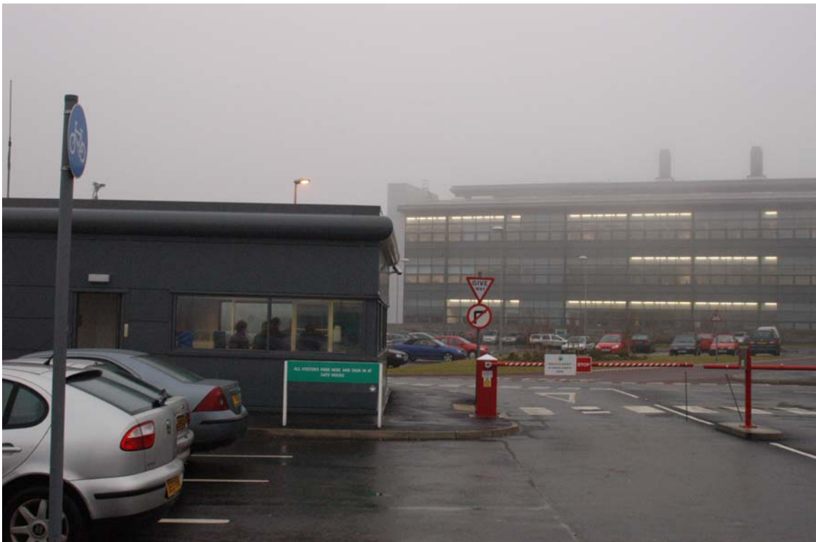
Photo 3 - Main Gate facility view
